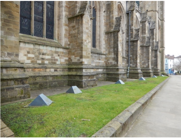
Low-key screened lighting fixtures...
