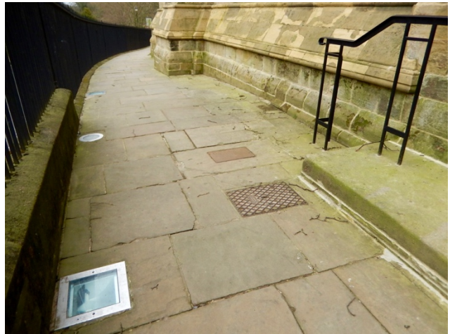
...or here built into the paving
